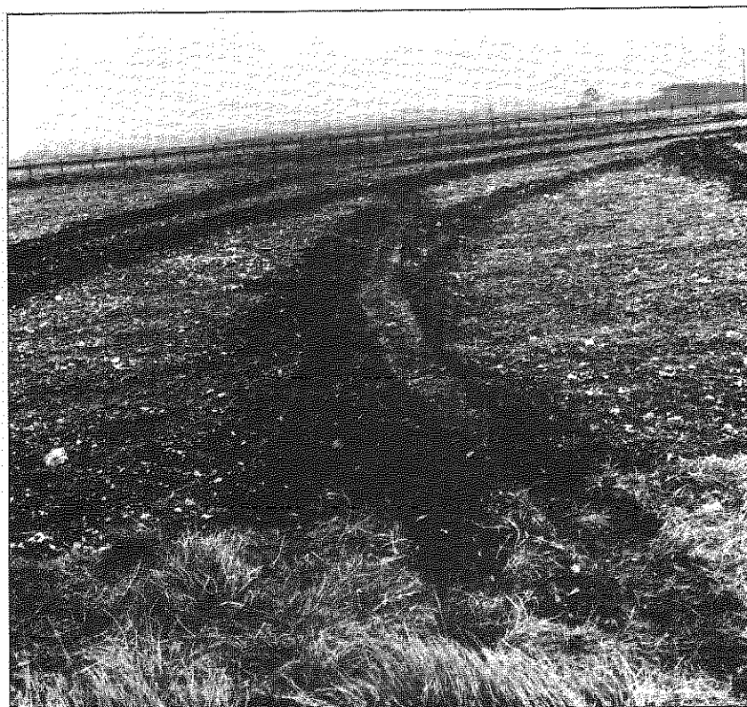
FIG. 29. A. & A.E.E. SOFT EARTH STRIP. RUTTING IN TURNING AREA. 2 INCH WET SOIL ON FROZEN SUBGRADE.
