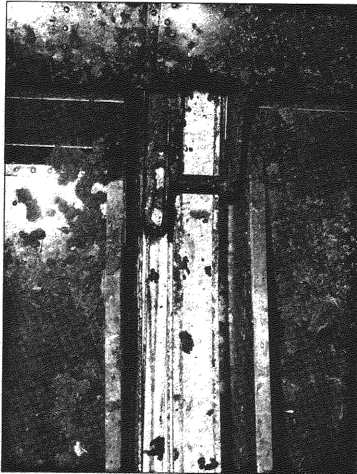
FIG. 22. CONTAMINATION OF FLAP TRACKS.
