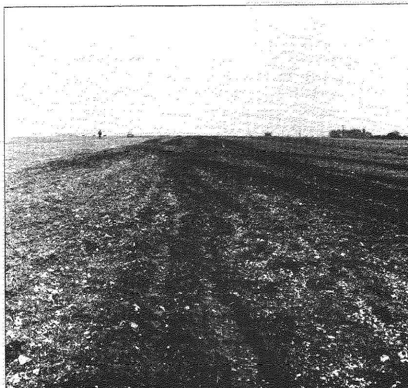
FIG. 28. A. & A.E.E. SOFT EARTH STRIP. RUTTING WITH SURFACE LAYER SOFTENED TO 3 INCHES.
