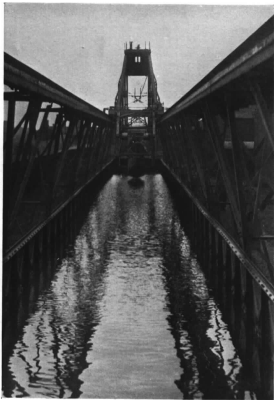
Looking towards the winch house.
